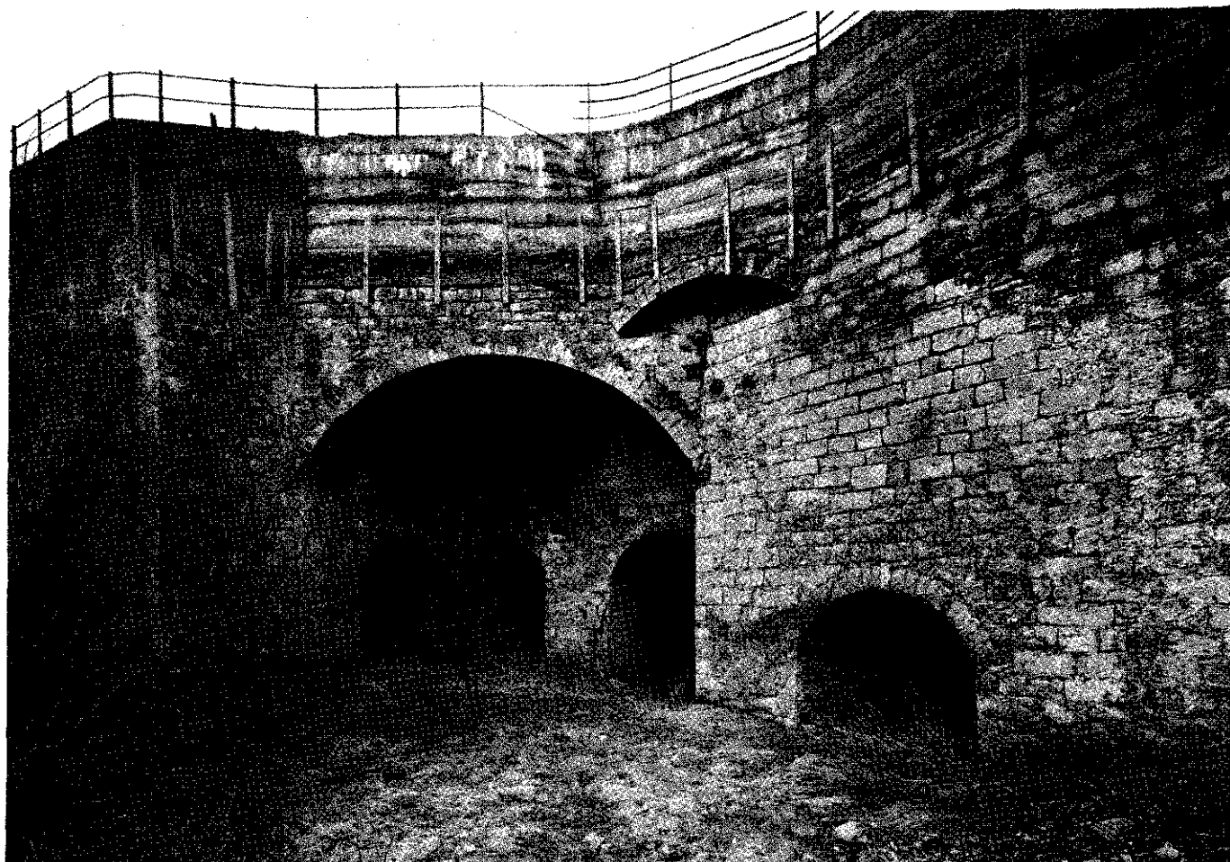
Illus 4. Roscobie Limekilns showing arched draw holes (A44303) (Copyright RCAHMS 1984).
